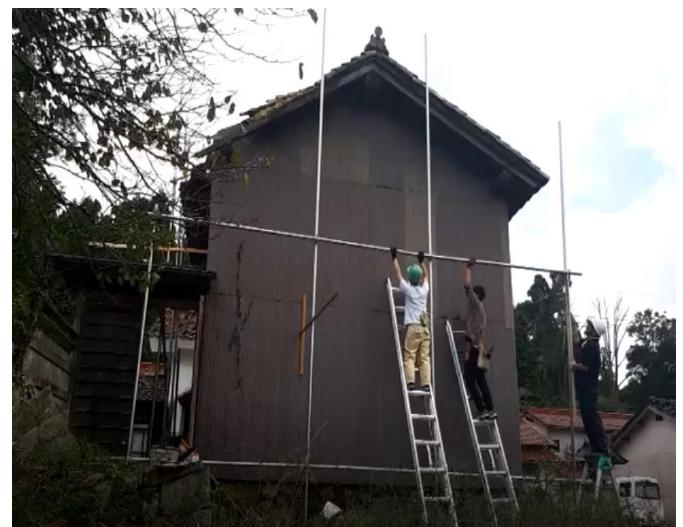
図3 作業風景 Figure 3 Work in progress
