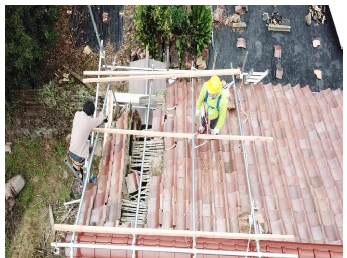
図4 作業風景 Figure 4 Work in progress
