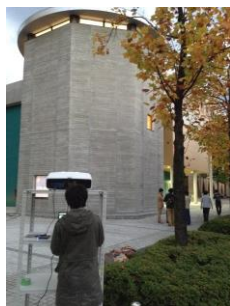
Fig.3 In our projection mapping, we selected this small gray concrete building as a target, depending on the capability of the projectors we have.
