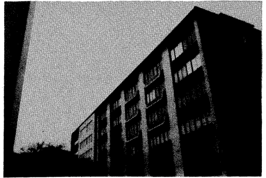
Fig. 7 Image of a building. The upper-right corner has three mutually perpendicular edges.
